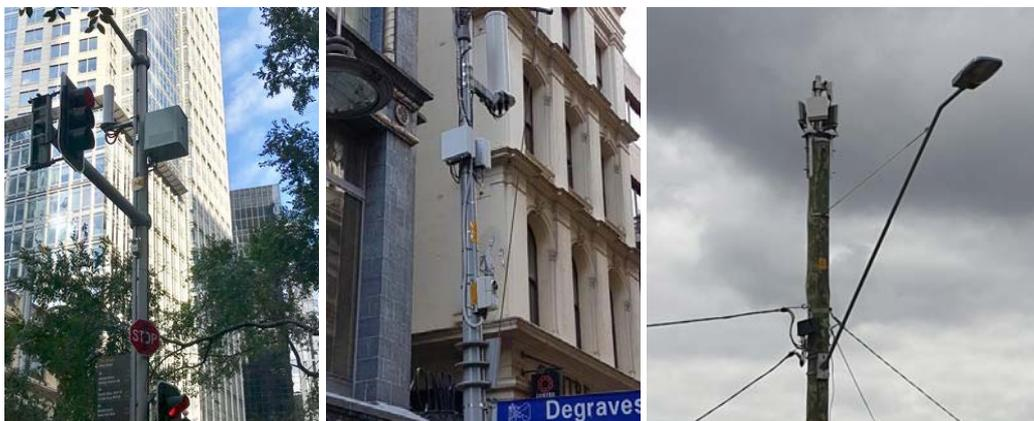
Figure 1: Typical Telstra Pole Mounted Small Cells
